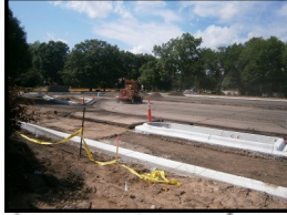
2015 New parking lot
