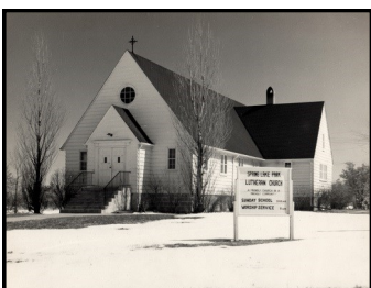
1940 First worship service held without doors or windows installed
