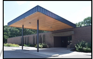
2019 "Open Arms" canopy completed
